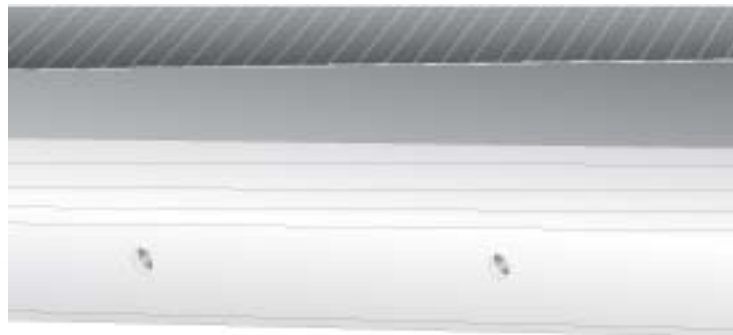
Image 4-24: Holes drilled for potential equalization
